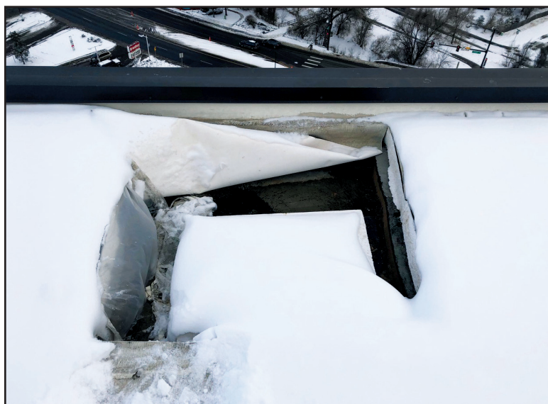
This damage occurred when a contractor failed to perform any repairs at areas of intrusive testing. Six similar cuts were made and not repaired. When a snow storm hit the building, these cuts were a significant source of water intrusion into a multifamily high-rise building in Denver.
