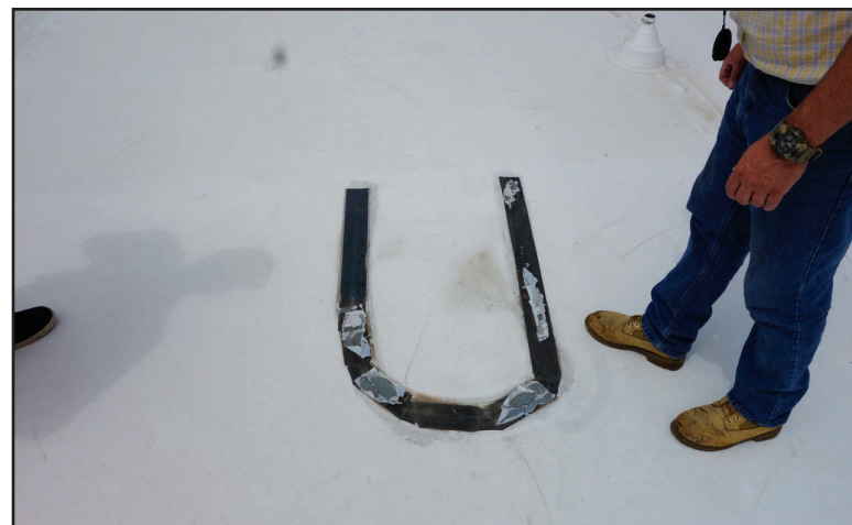
This repair was performed by a roofer selected by the insurance company. The repair used the wrong roof membrane material, was not repaired in accordance with accepted industry practices and was poorly executed, resulting in water intrusion into a building with high amounts of asbestos-containing materials. This type of mistake was made on nearly 20 buildings of a multifamily community.
